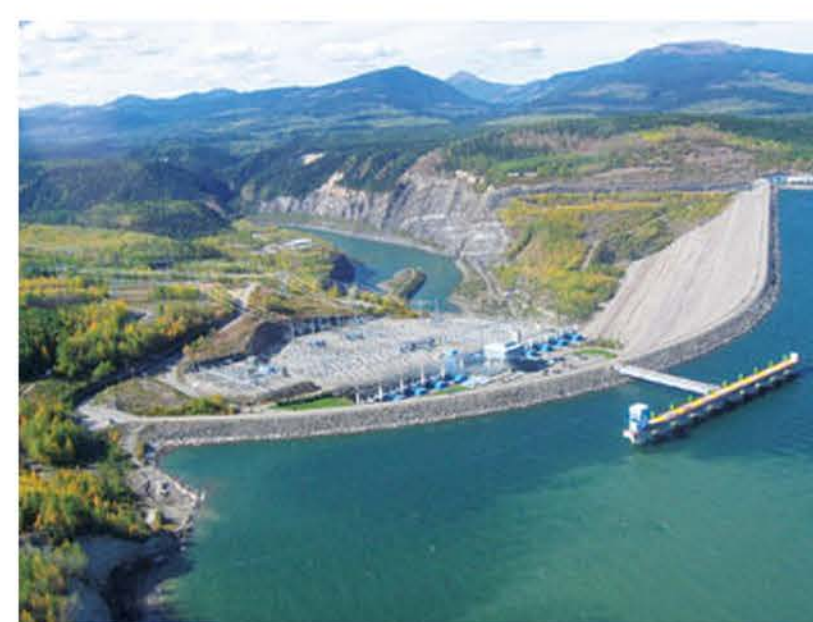
The Peace River Gordon Shrum Generating Station
