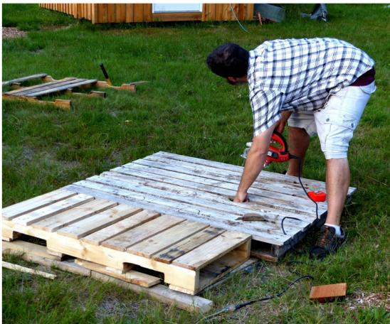
Cutting holes for 4" PVC tubes that create 6 air channels into the compost pile.
