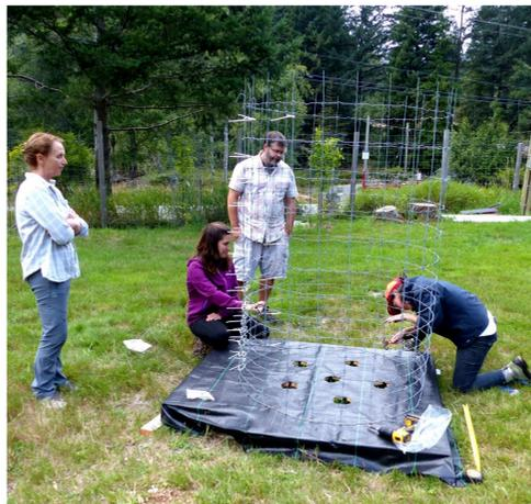
Attaching the wire frame to pallet. The 6 holes will hold the PVC pipes.
